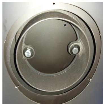
2.) Unscrew the 2 x M8 bolts in the inner rear flue pipe panel and remove the panel
