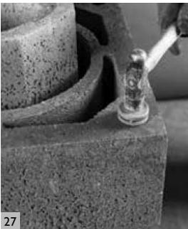
At the top of the chimney, insert capping fixings into the four corner holes of the casing
