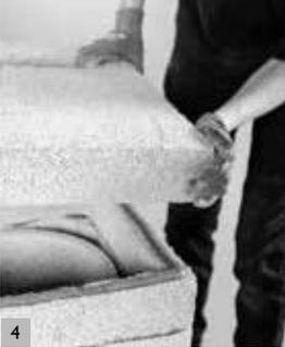
Apply glue to the whole surface of the block before placing the stove recess baseplate.
