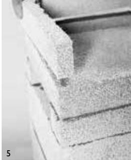
Apply glue all around the edge, with the exception of the front edge where the appliance will be fitted.
