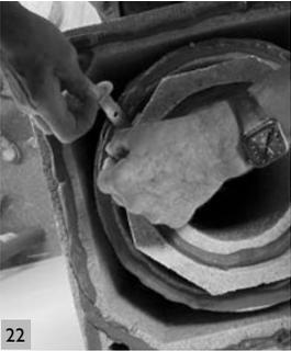
22 4x steel spacers push fitted around inner flue block every 1m of chimney.
