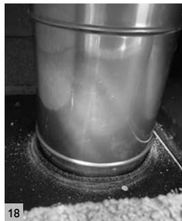
The steel pipe is sealed into the stove using fire cement.
