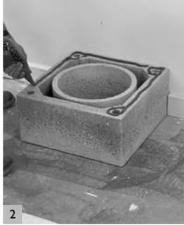
Apply glue to the whole top surface of the module before placing the the next block.
