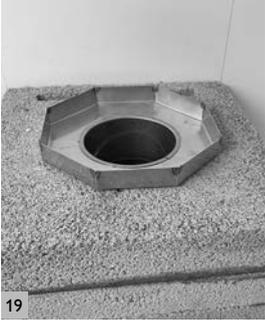
19 The Octagonal stainless steel adaptor slides down inside the stainless steel pipe shown previously. The bottom of the Octagonal adaptor lies flush onto the Pumice top plate.
