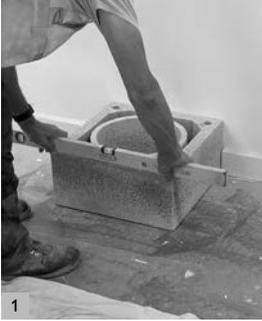
Measure and note the desired location of ISOKERN CELSIUS solution. Apply Schiedel ISOKERN chimney glue to the pre-prepared load bearing reinforced concrete slab and place first pumice block. Use a spirit level to ensure that the block is positioned correctly, then the whole installation remains in level throughout its length.
