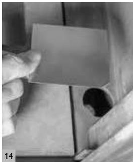
Remove the 2 thin cover plates, to get access to the adjustable feet (bolts) at the bottom. (IMPORTANT! Install the plates in position before the bottom vermiculite panels are reassembled).
