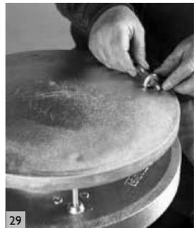
Fit aluminium top ring by pushing the steel prongs into the outside of the inner flue block.
