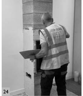
24 To finish off add render with reinforcement mesh being used up to ground floor ceiling.
