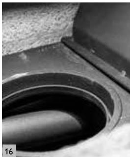
Putting your hand in through the top hole for the ventilation grill, pull the air inlet and flue pipe down into position. Glue is not required.
