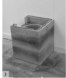
Apply glue to the module outer edge, with the exception of the gap for the first ventilation grill.
