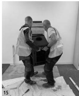
Now slide the appliance into position and adjust and fix using the 3 screws at the bottom.
