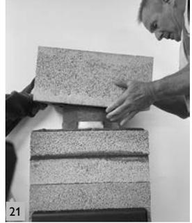
21 The first outer chimney block is glued into place, making sure it's square and level.
