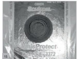
View of the finished vapour barrier sealed tightly all round.
