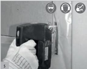
5 Make the opening. **NOTE: Load bearing elements must not be weakened!** **IMPORTANT: follow the safe working notes on page 31.**
