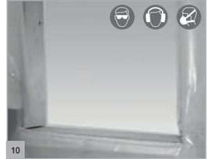
If necessary correct the opening. Replace the thermal insulation right around the assembly opening in the studwork. **IMPORTANT: follow the safe working notes on page 29.**
