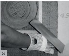
Check that the thermal insulation is flush with the wall.
