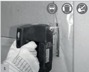
5 Make the opening. **NOTE: Load Bearing elements must not be weakened! IMPORTANT: follow the safe working notes on p.35.**
