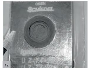
Insert Ignis-Protect so that it fits perfectly. The side laminated with foil should be facing inwards!
