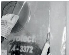
With Ignis-Protect in place, cut away the vapour barrier flush to the edges.
