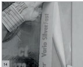
Secure the junctions with the vapour barrier by applying appropriate sealing tape to the foil lamination.
