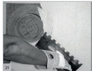
Application of render over the whole surface. **NOTE:** do not render over the inner protection pipe!
