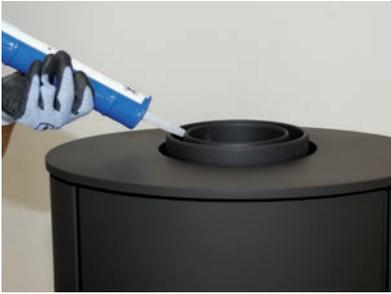
1. Make sure the outlet on the stove is installed correctly, according to the installation manual for the stove. Apply high temperature liquid sealant on the inner and outer ring of the stove outlet to provide a gas tight connection.
