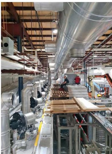
A recent project for Dijke Ovens saw a custom built concentric system specifically for the oven types designed by Dijke. Approximately 6% of the heat is recovered and used to supply heat back into the ovens, making the system exceptionally efficient.
