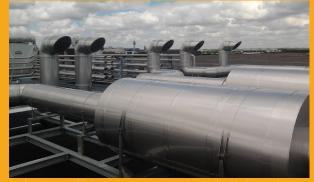
In this picture: High pressure system solution (incl. silencers)
